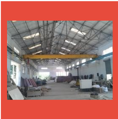
Over Head Crane
