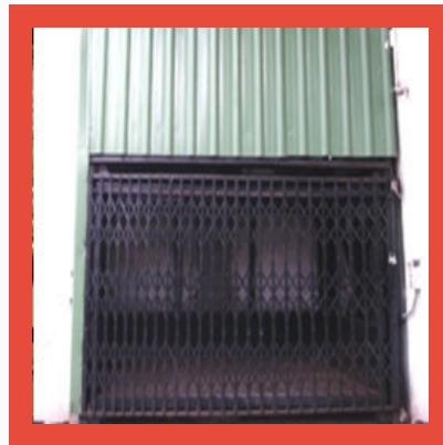
Material Handling Goods Lift
